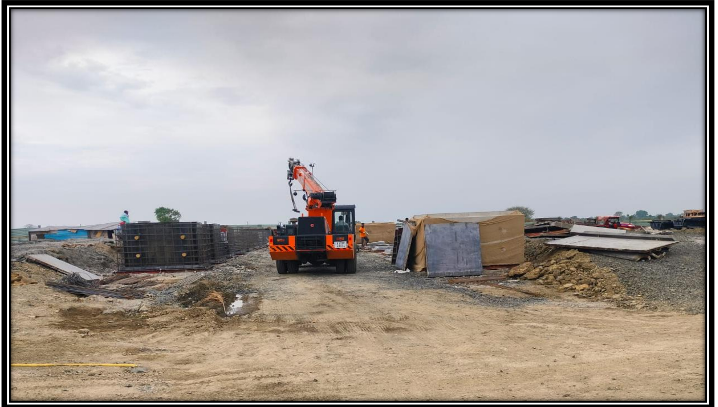
Box Culvert Segment Casting work in Progress at Km 107+500
