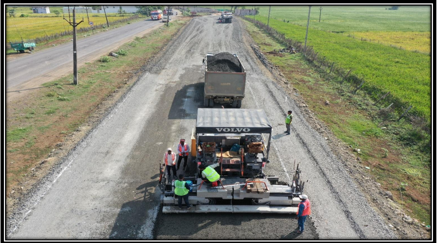
CTB Laying in progress
