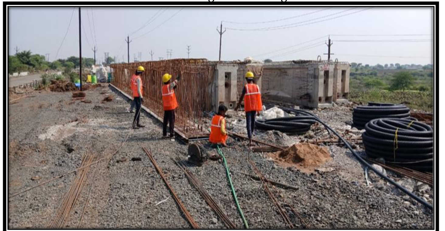
Girder Casting Work in Progress
