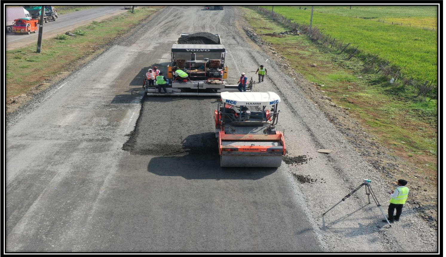
CTB Laying in progress
