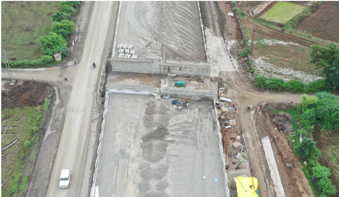
Work in progress at Km. 105+268 LVUP
