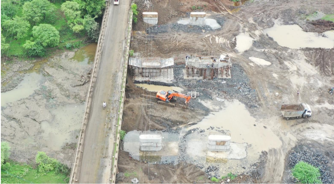
Work in progress at Km. 109+544 MJB
