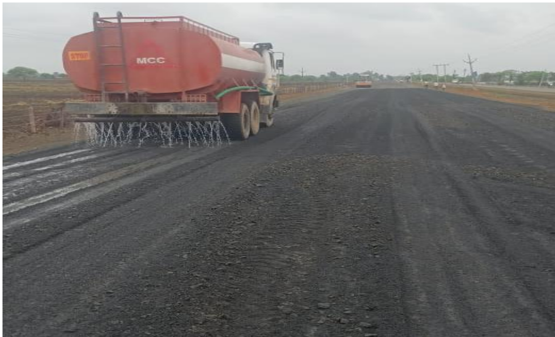
GSB Work in progress at Km. 121+780 to 121+960
