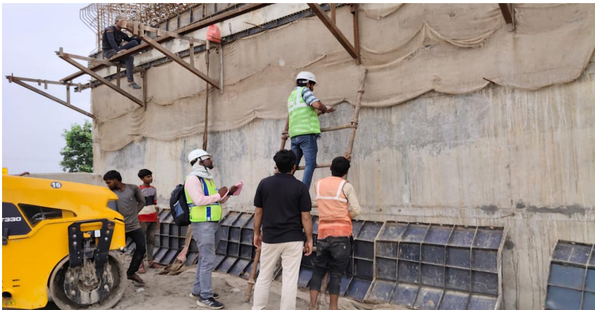
NDT Test Work in progress at Km. 113+575 VUP
