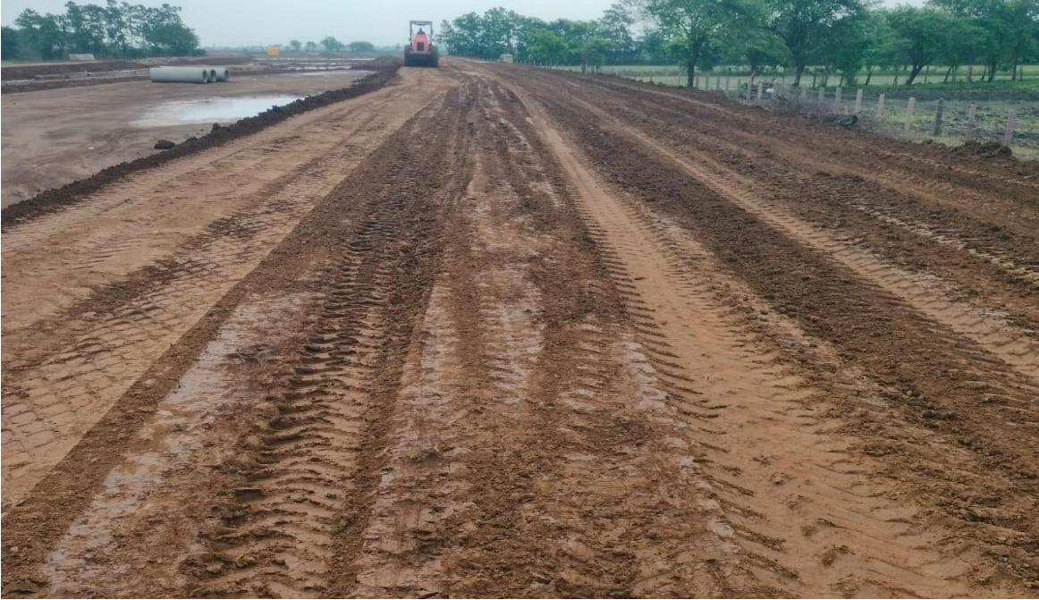
EMB Work in progress at Km. 125+000 to 125+300
