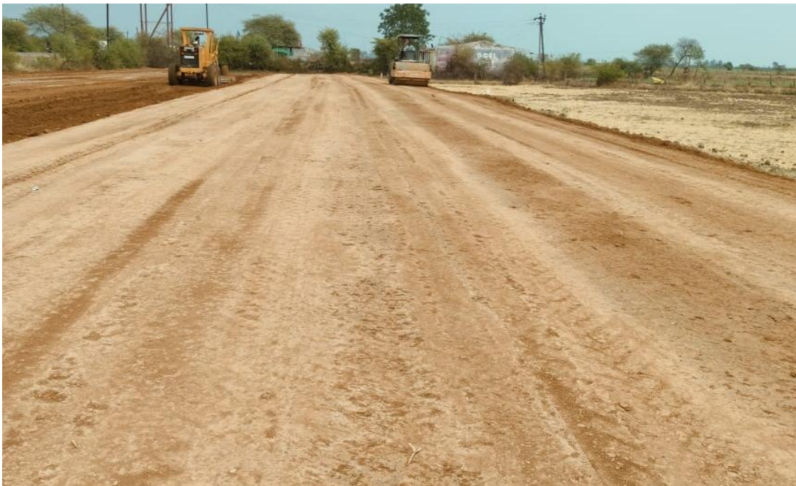
EMB Work in progress at Km. 122+900 to 123+150
