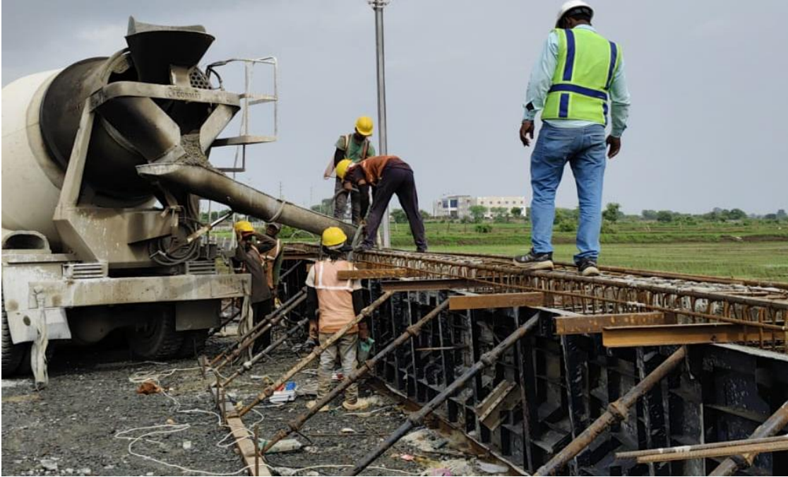
Girder Casting work in progress at Km. 109+500
