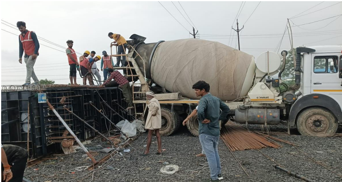
Girder Casting work in progress at Km. 109+500
