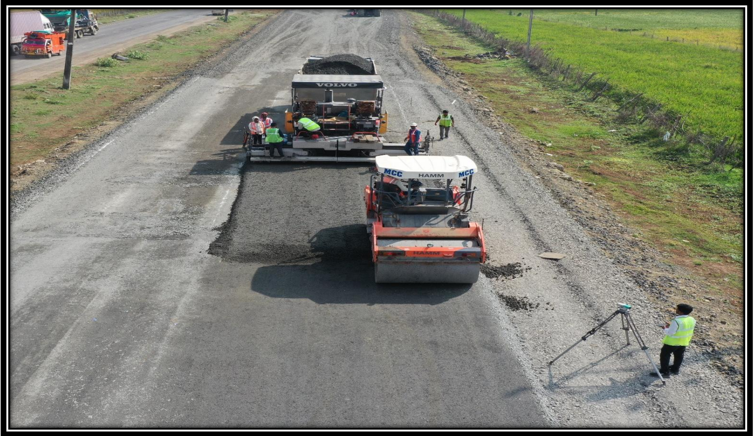
CTB Laying in progress
