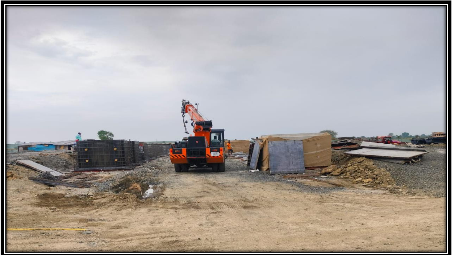
Box Culvert Segment Casting work in Progress at Km 107+500
