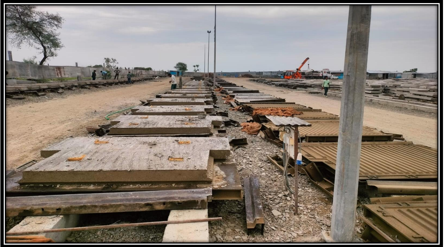
RE Panel Casting work in Progress at Km 107+500
