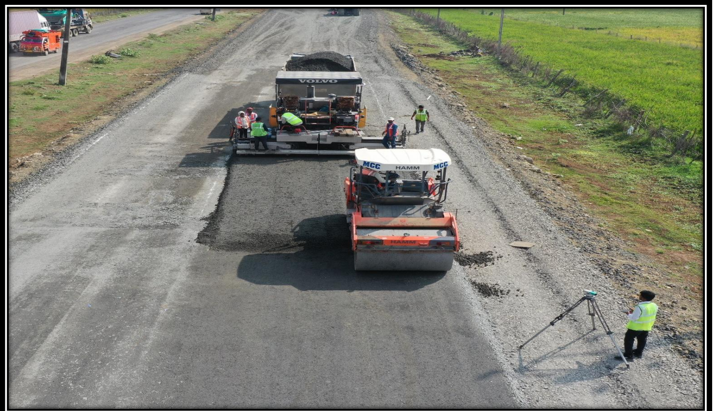
CTB Laying in progress
