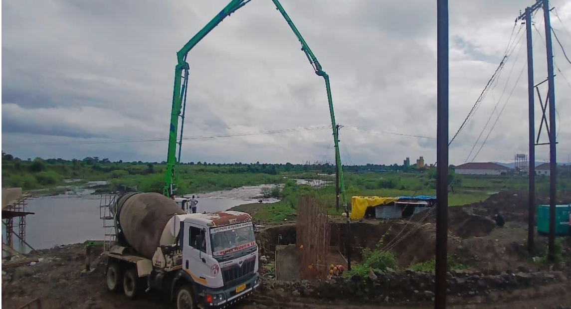
Girder Casting Work in Progress
