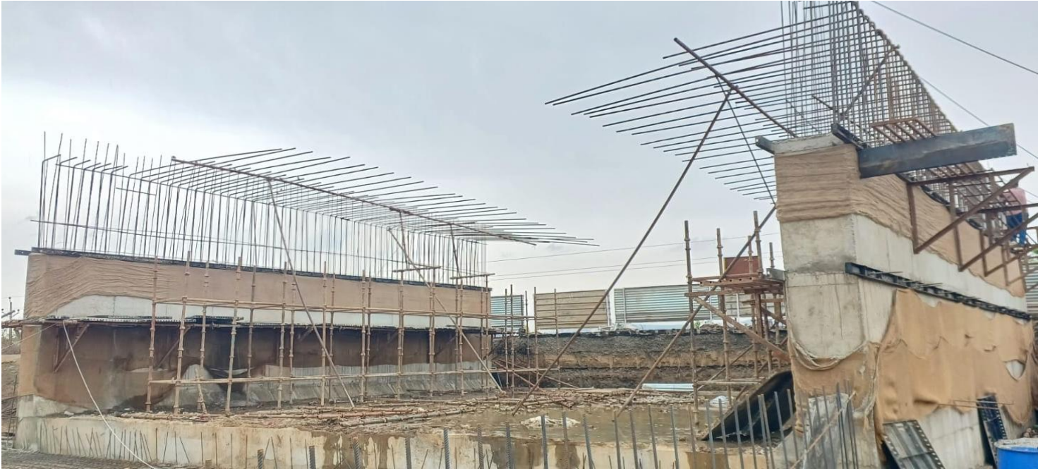
LVUP work in Progress at Km 105+280
