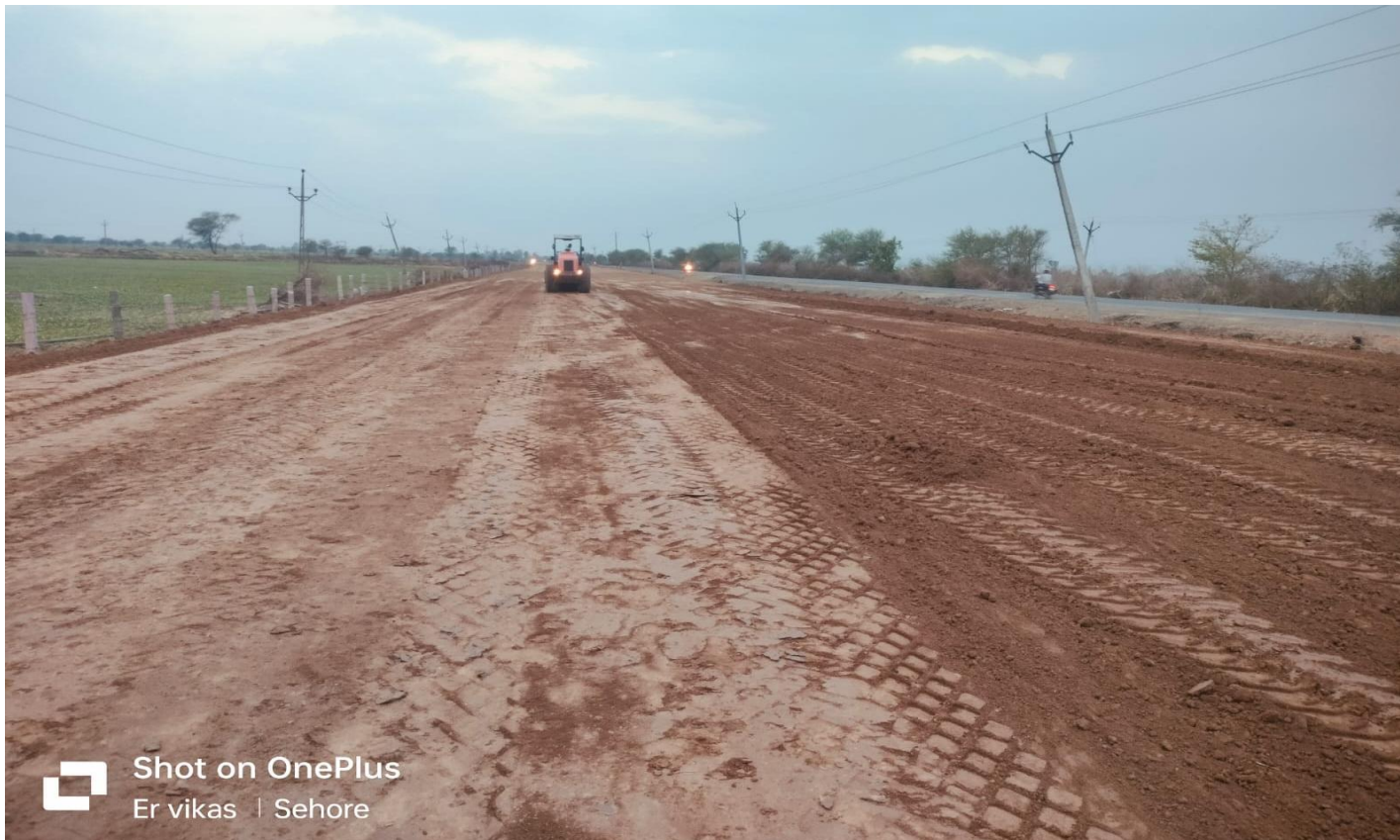
EMB Work in progress at Km. 122+140
