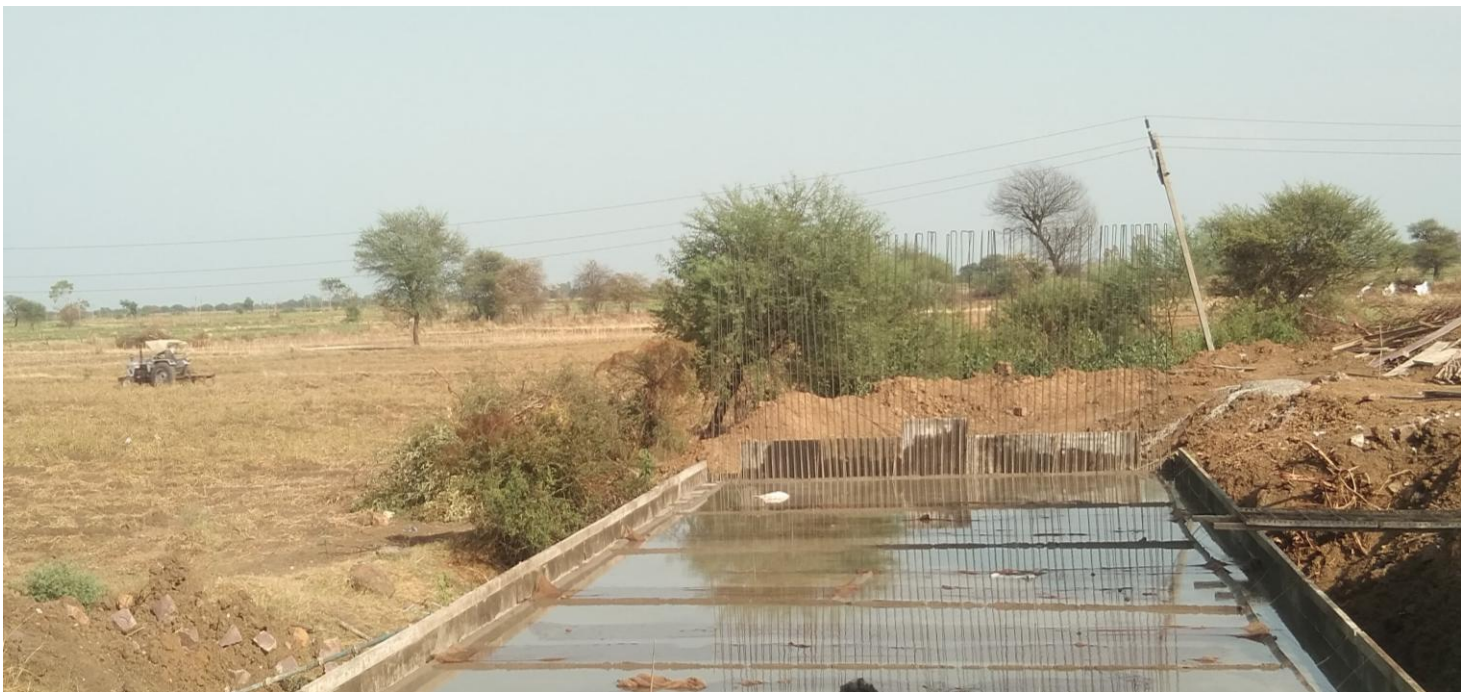
MNB work in progress at Km 123+222
