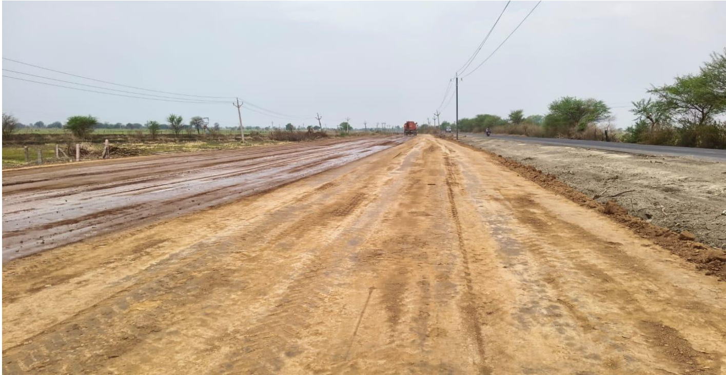
EMB Work in progress at Km. 140+320
