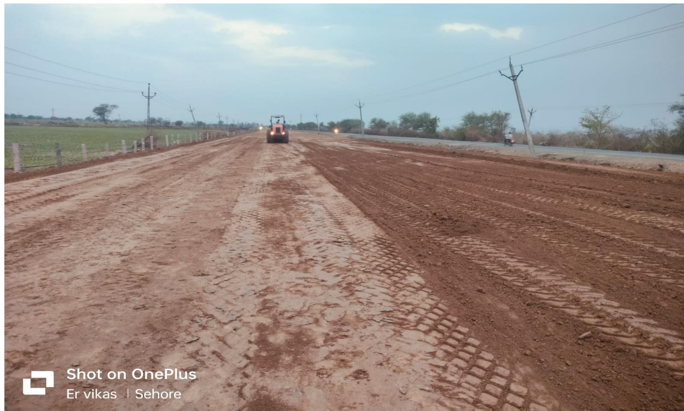
EMB Work in progress at Km. 122+140
