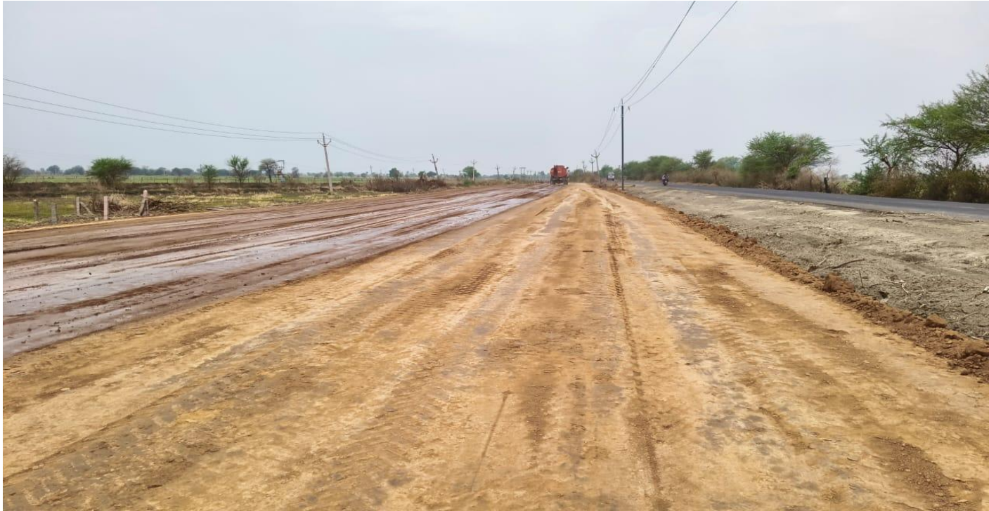
EMB Work in progress at Km. 140+320
